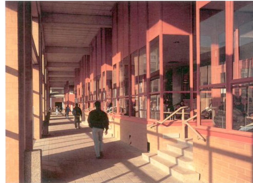
Figure 6.1: York University Student Union- a weather protected walkway flanks the building at the ground floor. Rolling garage doors can be opened during summer months to provide an open colonnade
