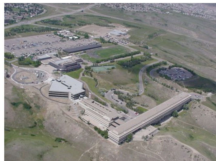
Figure 1.2: Aerial view of the campus
