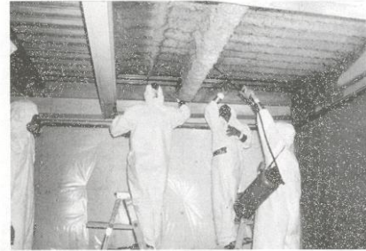
Typical high risk abatement project
